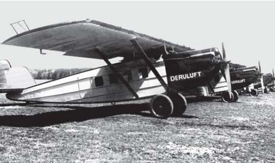
A Dornier Merkur aircraft from the pioneering German-Soviet airline powered by a BMW VI aero-engine.
