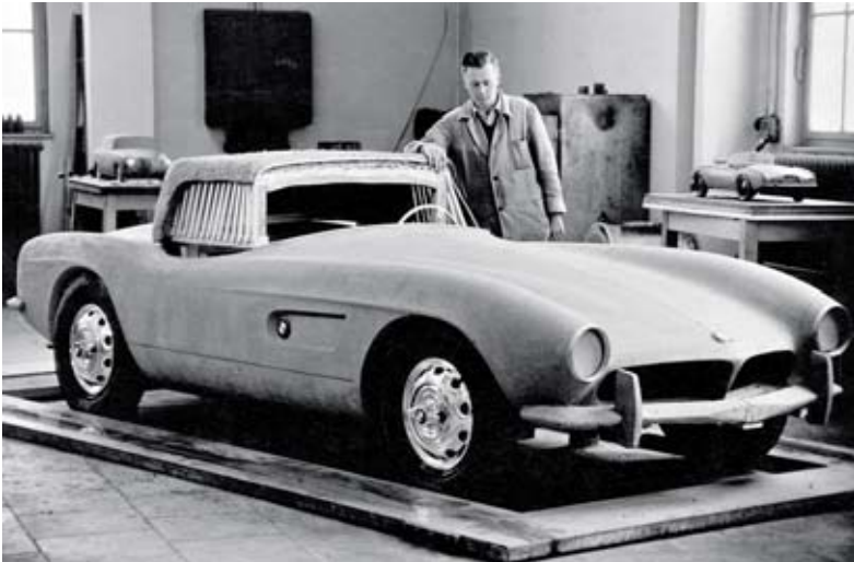
BMW model builder Johann König in 1954, working on a clay model of the BMW 507.
